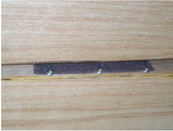
thick wire spring extenders with felt vibration damper
